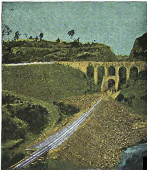
AQUEDUCT OF JALAPA.
